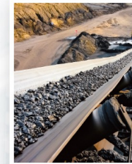
Mine Belt Conveyor
